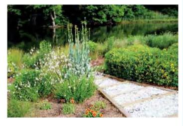
When parking lot run off created a problem, the Master Gardeners turned it into a feature. Stairs filled with stone and soil allow storm water to drain and filter before eventually entering the creek. Photo courtesy of Northern **Neck Master Gardeners**
