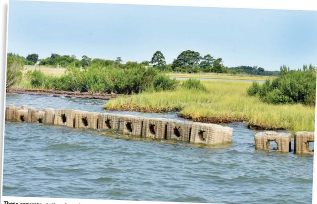
These concrete stations have been placed near marshes south of Hogg Island in the York River to protect the island from erosion. Photo by Larry Chowning
