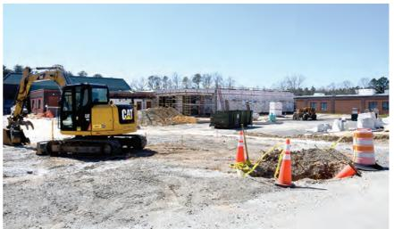
Renovations and additions at Lancaster Middle School, 191 School Street, Kilmarnock are ongoing as the facility is converted into an elementary school. The project includes demolition of a 1960s classroom wing and construction of an approximately 7,700-square-foot addition for a new main entrance, administrative suite and new classrooms. The renovation scope covers 66,000 square feet. Photo by Lisa Hinton-Valdrichi
