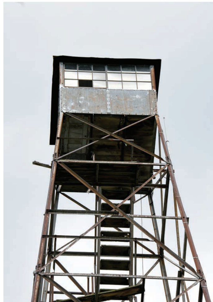
The cab on the Miskimon Fire Tower shows years of wear with broken windows and rust. Photo by Lisa Hinton-Valdrighi
