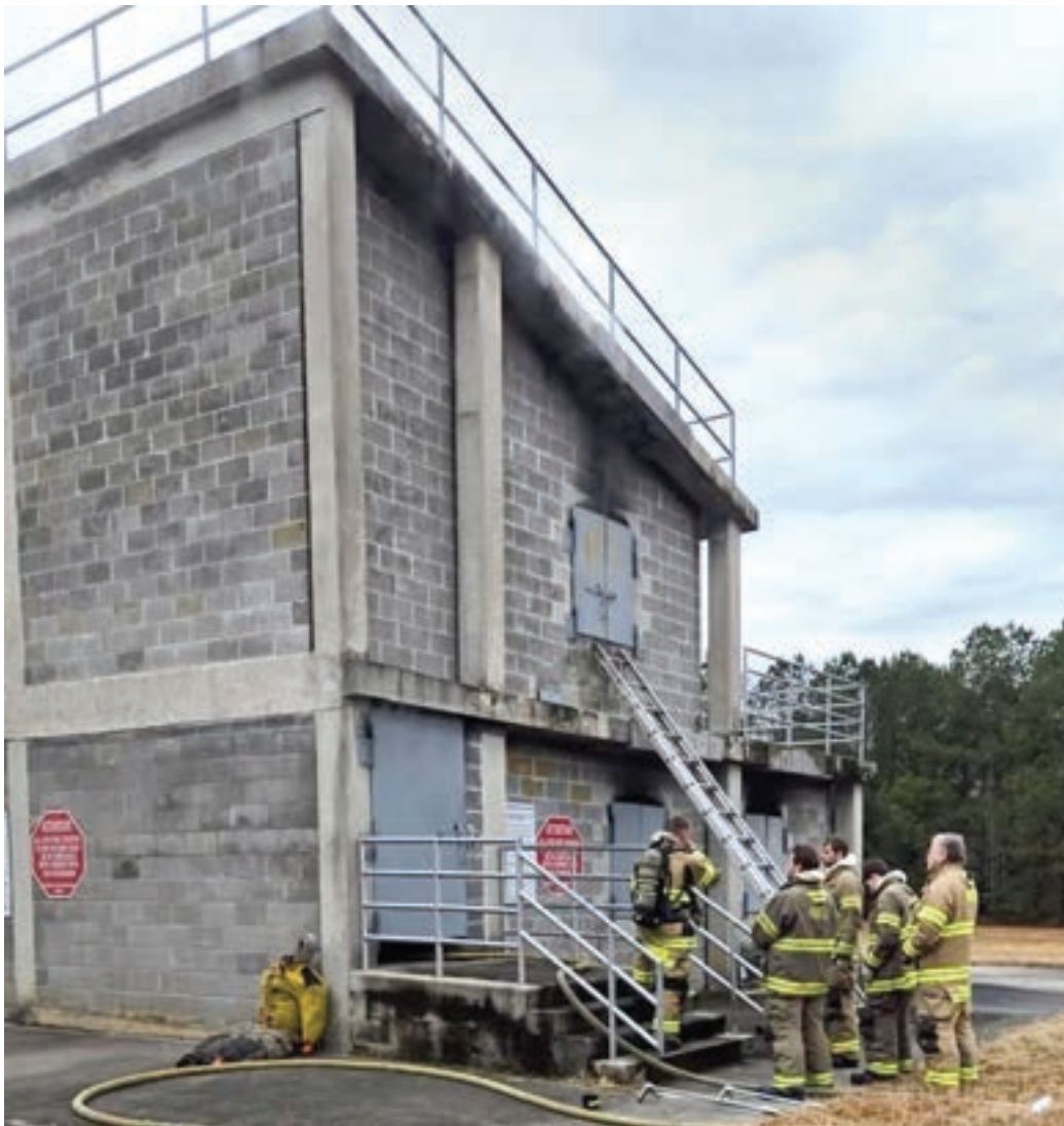
The burn building in Browns Store serves as a regional training facility for volunteers in Northumberland, Lancaster, Richmond, Westmoreland and Essex counties. Photo courtesy of Kilmarnock Volunteer Fire Department
