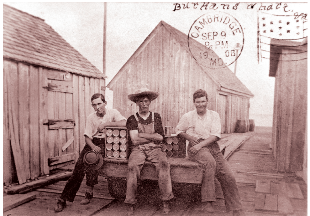
Burhan’s Steamboat Wharf at Locust Hill had a post office named Cooper. A pickle factory was also located on shore where local farmers sold cucumbers and were paid so much for each basket of 100 cucumbers. The rail car carried cans and freight from the end of the wharf to shore. The wharf was named after John S. Burhan of New Jersey who built the wharf in 1887. Courtesy of the late Jack Miller
